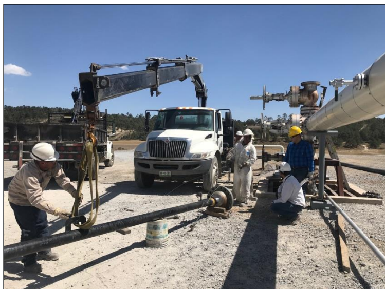
Figure 7. Preparations at well head for lowering the hexagonal sample holder with samples downhole. Pictures from CFE.
