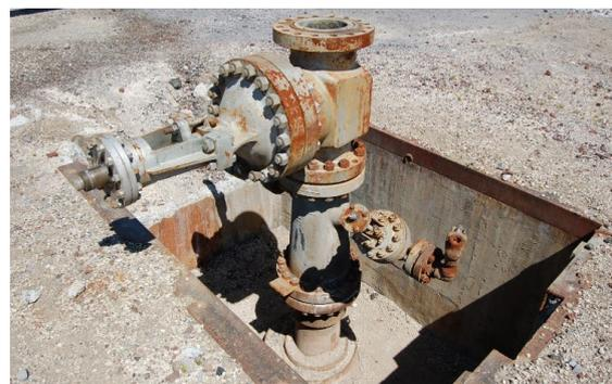
Figure 12: (Left) Hexagonal bar with test specimens which is lowered into well H-64 in Los Humeros. (Right) Well head of the H-43 high-temperature well in the Los Humeros geothermal field (Kruszewski & Wittig, 2018).
